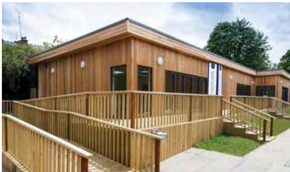
Upgraded "temporary" warming house example with permanent foundation (Minneapolis Park and Recreation Board)
