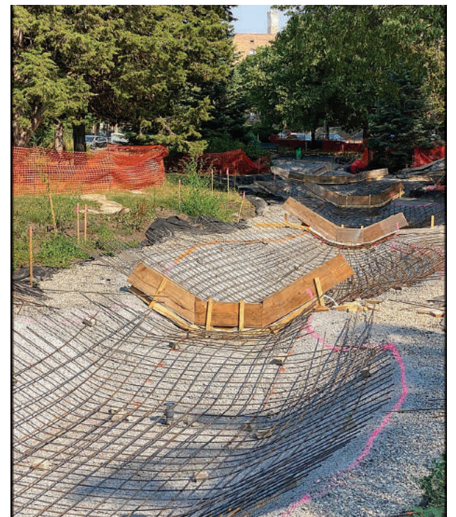
7 Pools reconstruction photos
