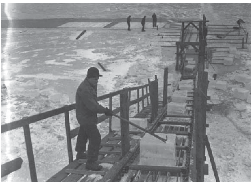
Conveyor belt moving ice cubes from Cedar Lake, 1948.
