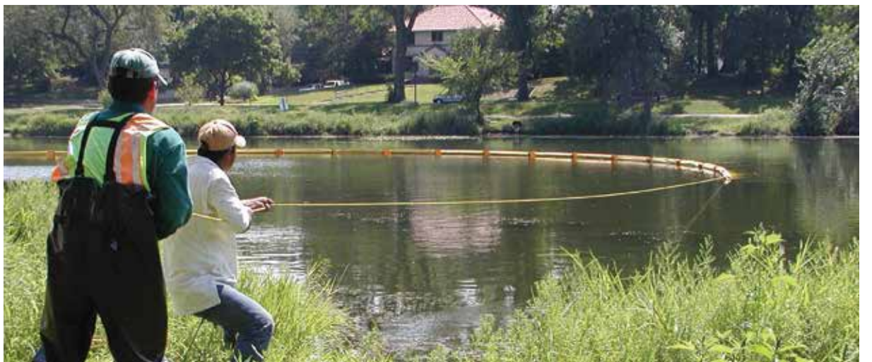
Setting the boom for Lake of the Isles renovation 2001
