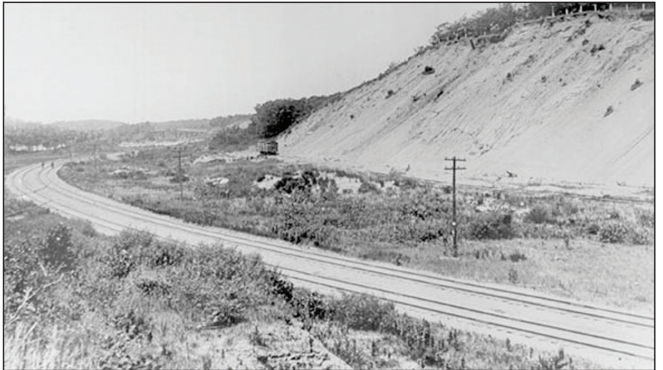
William Wallof. New Great Northern Railway Tracks at the base of the Bryn Mawr Bluffs, 1900s. Courtesy Minneapolis Collection, Hennepin County Public Library.
