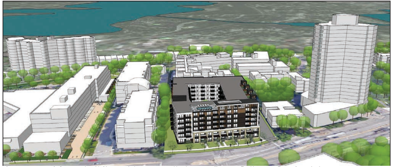
6-story wood frame building with west wall close to Loop-Calhoun Condominiums
