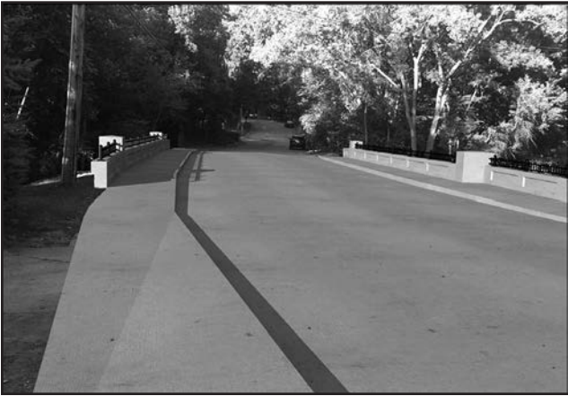
Artist's rendering of new bridge shows picket fence-style railings and six-foot-wide sidewalks (an improvement over the current five-foot-wide sidewalks).
