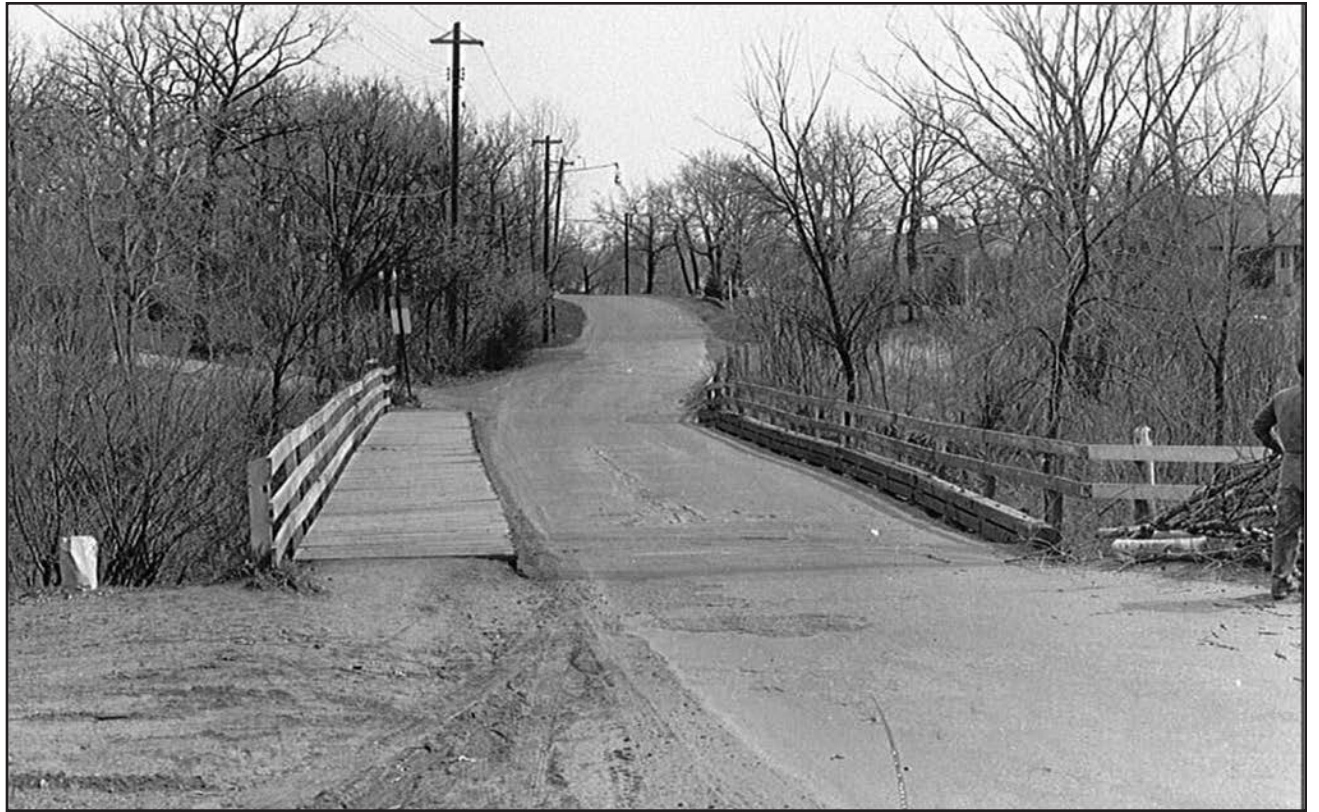
The first Burnham Road bridge over the Kenilworth Channel, shown here in April, 1961, just before its dismantling, was built in the 1920s through what was then a sparsely populated, bucolic corner of the city. (Photo courtesy Kent Madsen, Department of Public Works bridge inspector)
