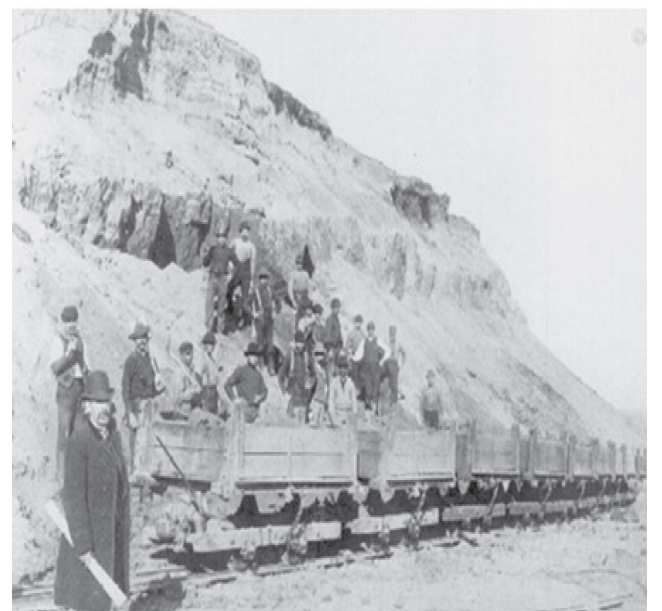
Here is a photo of the excavation of the Devil's Backbone from 1886. To give you a sense of how much fill was removed from the ridge, the present-day elevation of the roof tops of the Burch Building and Belmont Apartments—across from Sebastian Joe's on Franklin—are roughly the height of the former ridge. The excavation made it not only possible to develop Lowry Hill but to expand the Minneapolis Street Railway Company, also owned by Thomas Lowry. The streetcar expansion linked Minneapolis with new "sub-urban style" residential developments to the Southwest.
