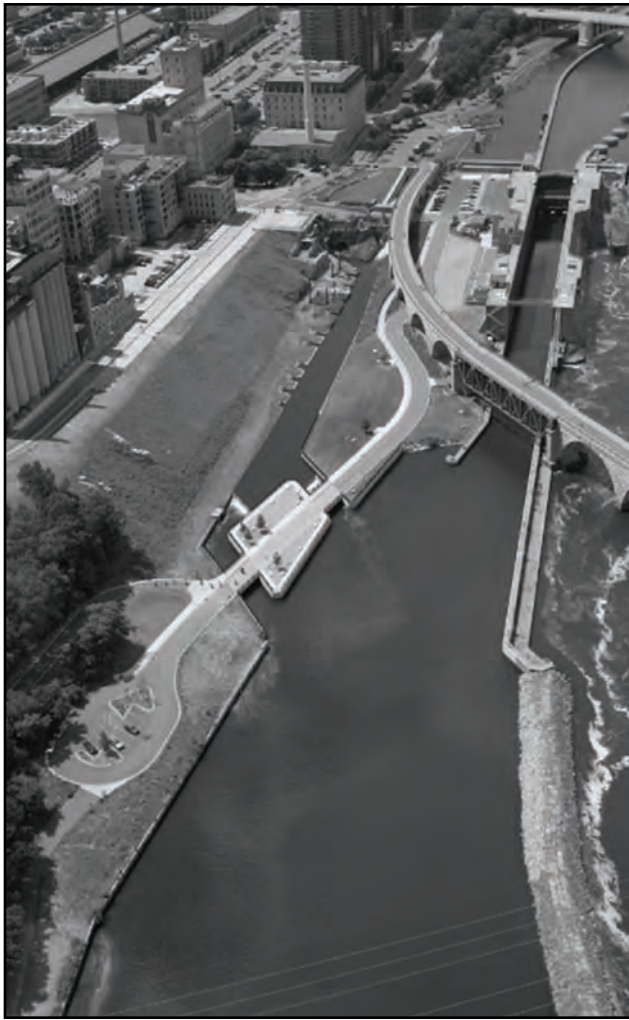
Water Works Site
