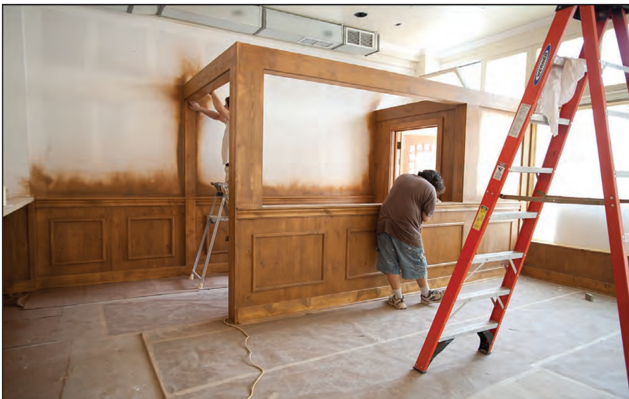
A sneak peak inside at renovations being done at The Kenwood.
