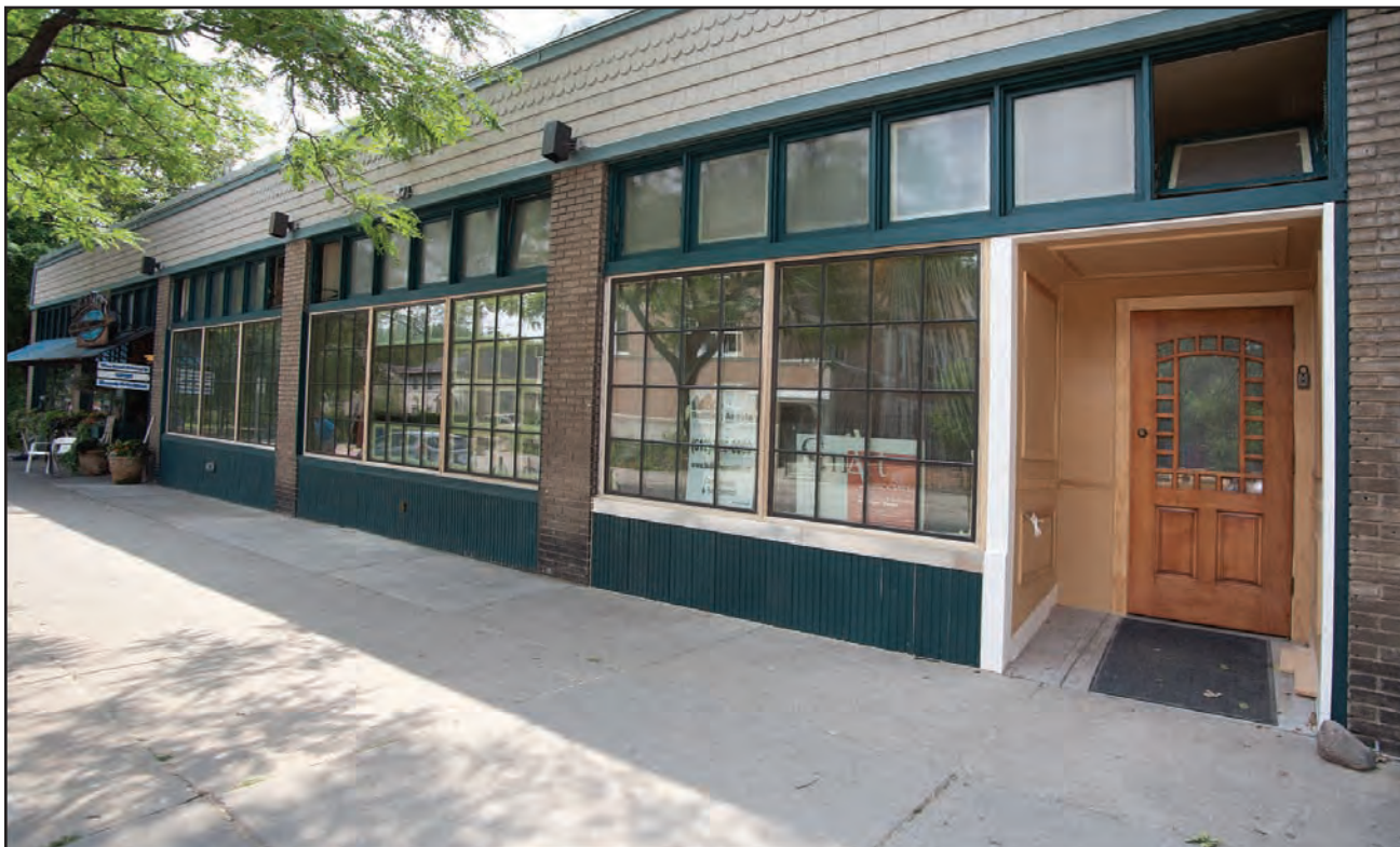
The Kenwood renovations are nearing completion.
