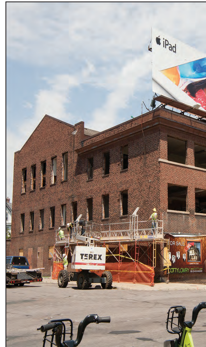
Renovation continues on the former Burch building Burch Restaurant.
